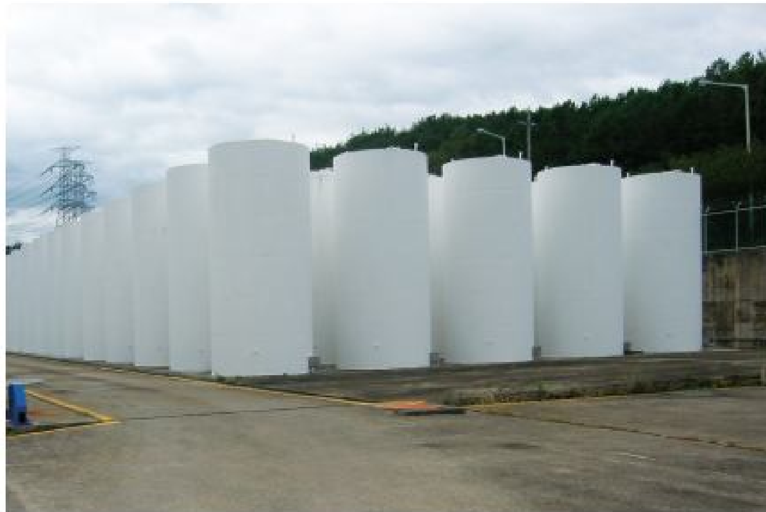
Figure 5.4 Dry concrete canister storage of spent nuclear fuel – Wolsong nuclear power plant, Republic of Korea. Eleven canisters are required to store the spent fuel discharged from one reactor over a year
